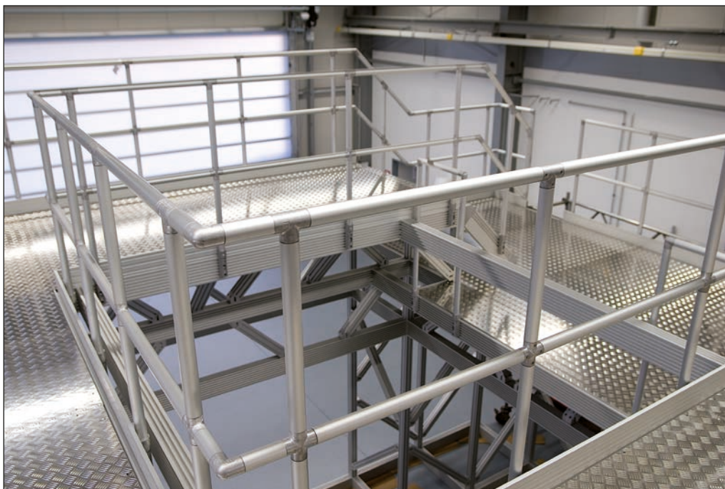
Working platform with ITAS railing
